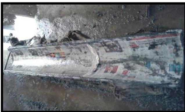
Fig. 4 Demoulding of Ferrocement Channel
