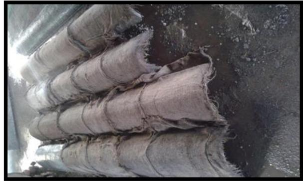
Fig. 5 Curing of Ferrocement Channels
