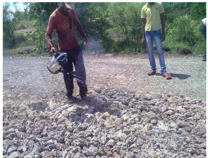
Fig. no.3- Bitumen spreading
