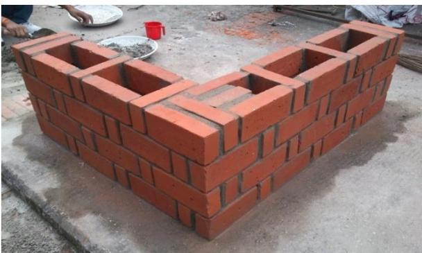
Fig.1 Typical picture of Rat-Trap bond
