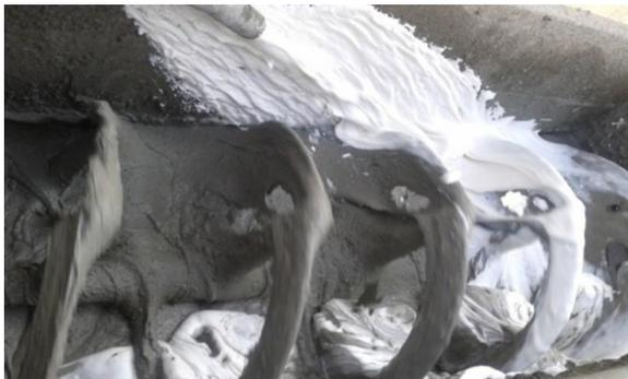
Fig. Mixing of CLC with foam
